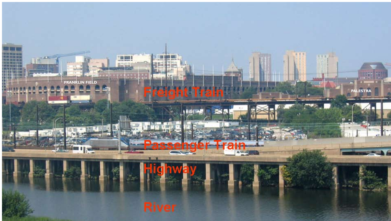
Photo of the east campus area as viewed from the east side of the river. The photo illustrates both the complexity of the infrastructure and the iconic quality of Franklin Field and the Palestra.
