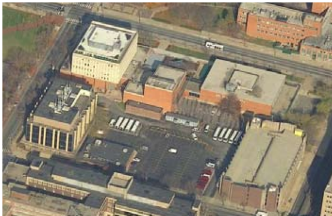
Existing Conditions at 3200 Walnut
