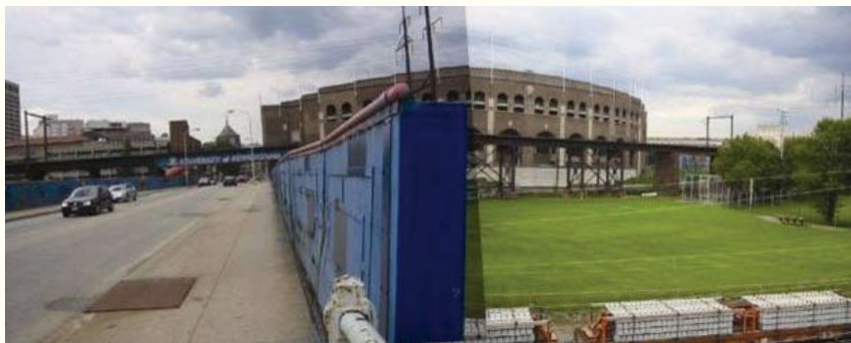
View of the South Street Bridge following reconstruction, illustrating the sports fields proposed on the top level of the South Street parking garage. The garage includes two floors of parking below the bridge level.
