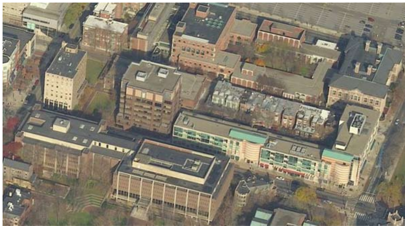
Existing Conditions at 3400 Walnut
