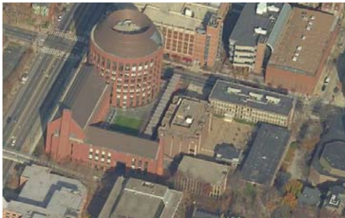
Existing Conditions at 3700 Walnut
